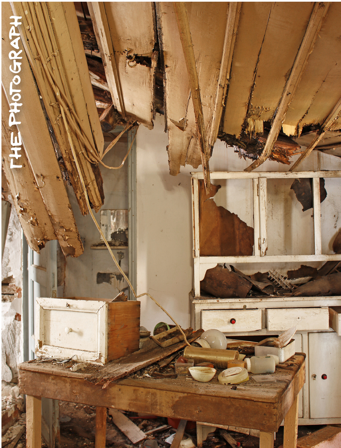
Kitchen in an abandoned 19th century house in Arcadia, Greece. Photo: Christoph Ziegler
